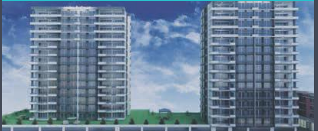
Uypa Residence Adana
